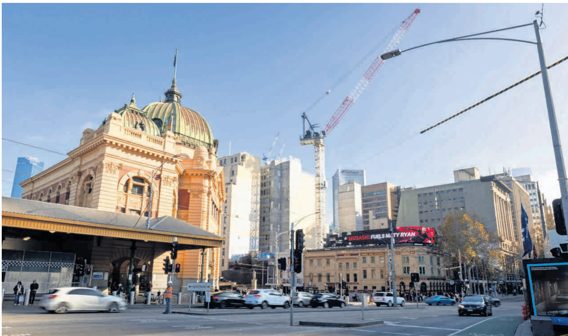
The proposed development would wrap around the Young & Jackson pub and potentially cast shadows over the neighbouring Flinders Street Station. Photo: Ruby Alexander
